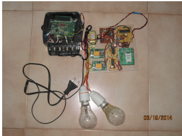
Fig. 6 Intelligent energy meter
